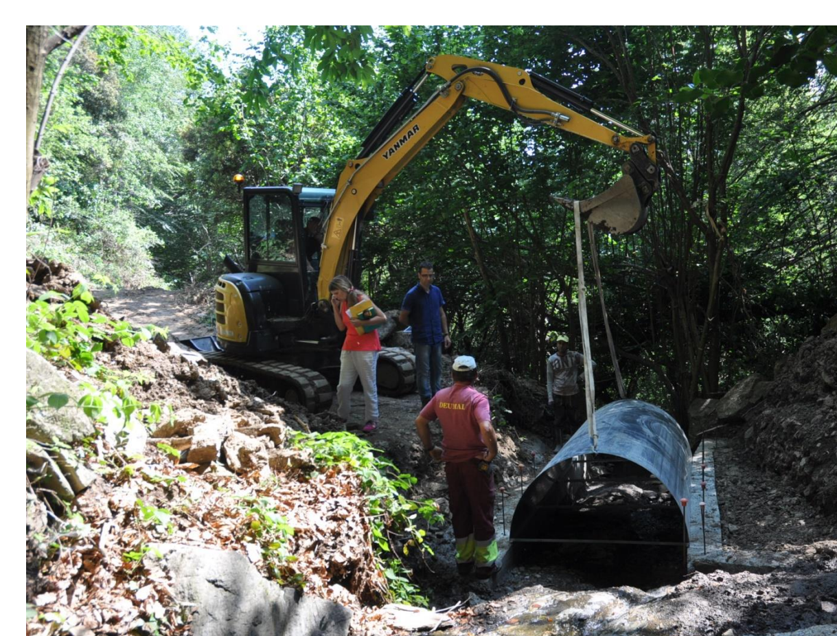
Vault installation in a stream
