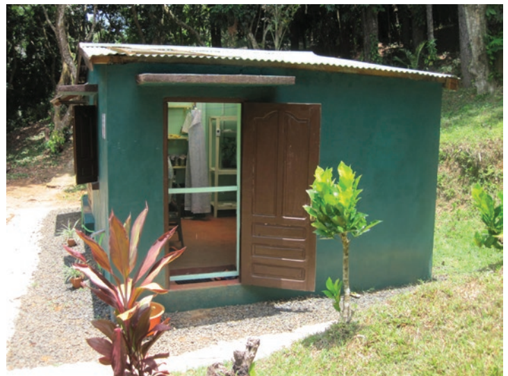
The new amphibian breeding facility at Parc Zoologique Ivoloïna. Funding from the AArk Seed Grant will be used to purchase supplies for the center, including a water treatment system, as part of enhanced biosecurity measures. Photo: Maya Moore.
