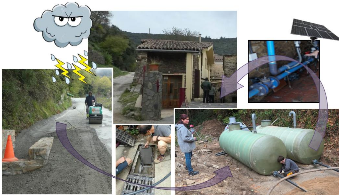
Rainwater harvesting cycle (collection, filtering, accumulation, pumping)
